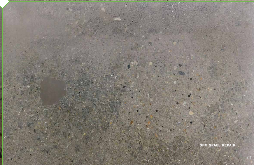
REPAIR WITH SRG AND EP80
